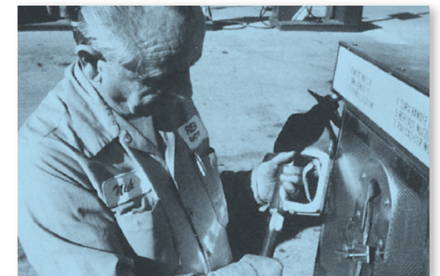
Inspect hose at the coupling for signs of leakage.
