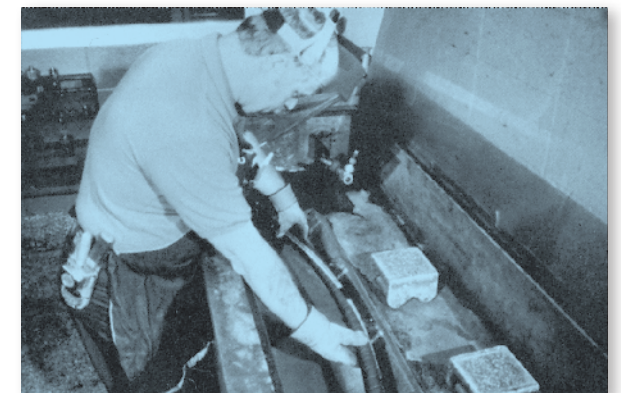
Hydrostatic hose testing.
